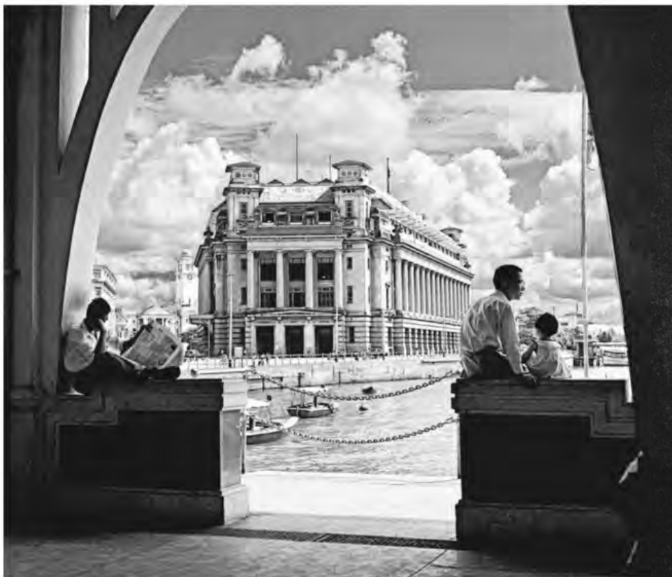
One of the highlights of the new book – Marjorie Doggett's Singapore: A Photographic Record – is this picture of Fullerton Building as seen from Clifford Pier, taken in 1957. PHOTOS: NATIONAL ARCHIVES OF SINGAPORE
